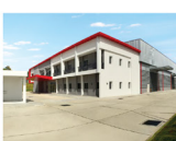
JUNE CHEWATHAI READY BUILT FACTORIES (2)
